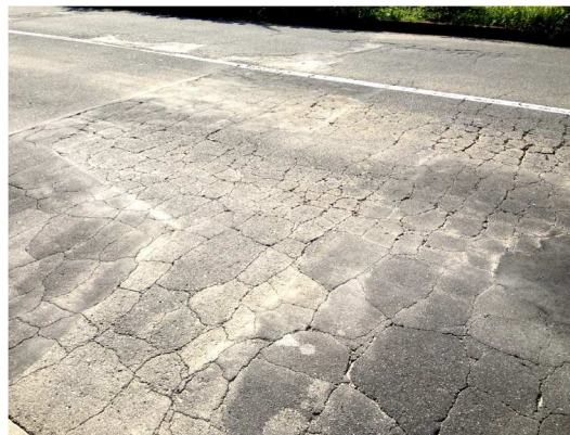
103 Figure 6. Target cracking of alligator cracking
