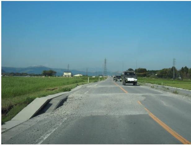
Figure 12. Bump step and pavement peeling at Aso City
