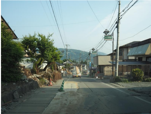
Figure 10. Pavement peeling at Mashiki Town
